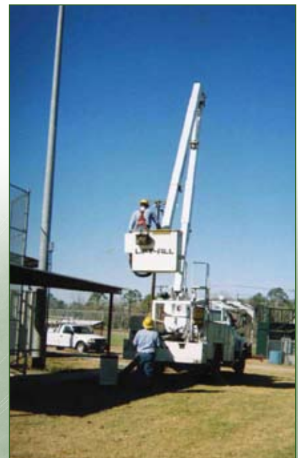
Crews repair damage to baseball and softball field lighting after Hurricane Rita.
